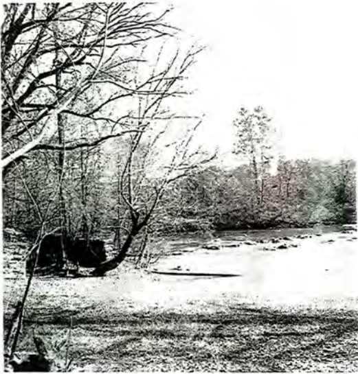
A. 9Mg99, Parks Mill. Mill foundation and dam from Southwest.
