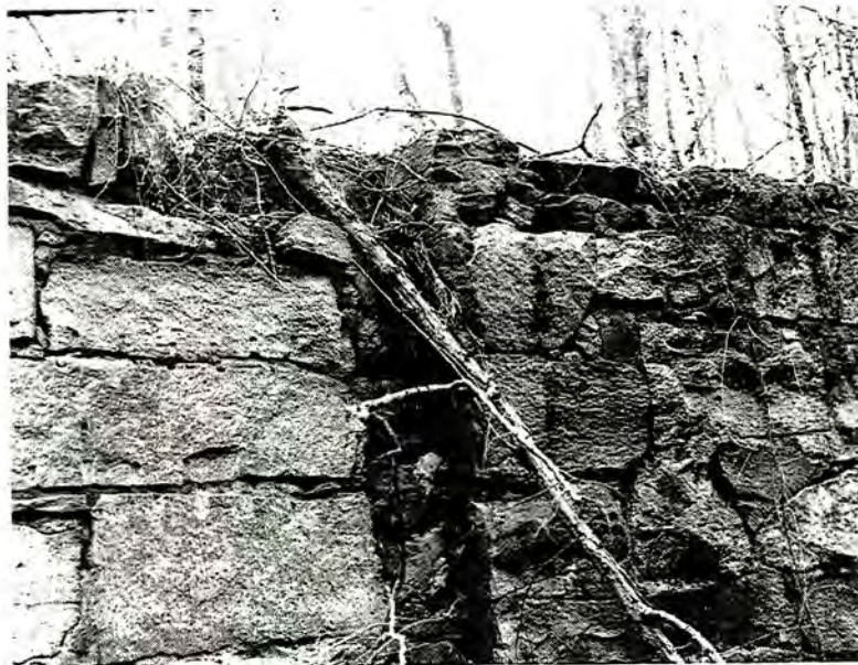
B. 9Ge37. Gate guide in North diversion gate from Southeast.
