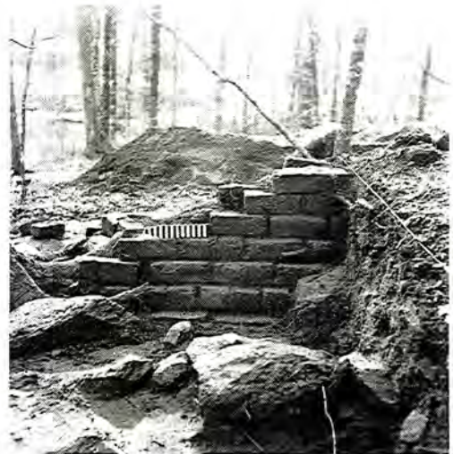
B. 9Ge37. Domestic structure 4 chimney foundation from Southeast. Scale in centimeters.
