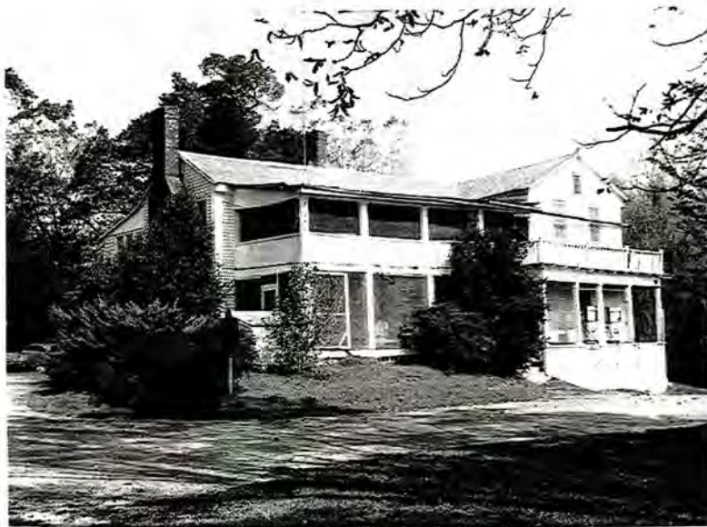
C. 9Mg99. Parks Mill house from Southwest.
