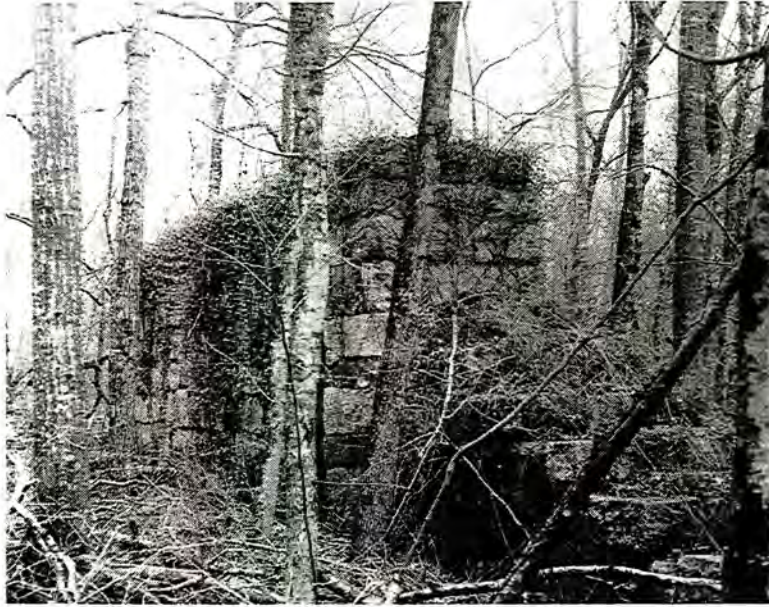
A. 9Ge37. South diversion gate from West.
