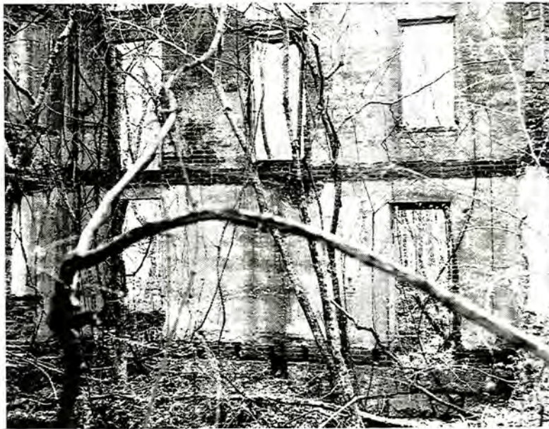
B. 9Ge37. Main factory building eastern addition. Interior plastered wall from East.
