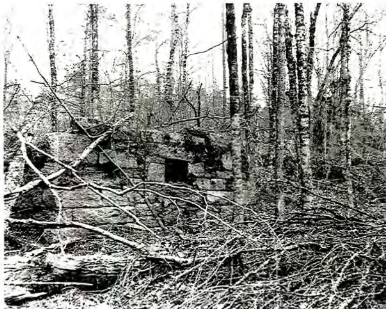
B. 9Ge37. Granite foundation of secondary mill building (str. 38) from West.
