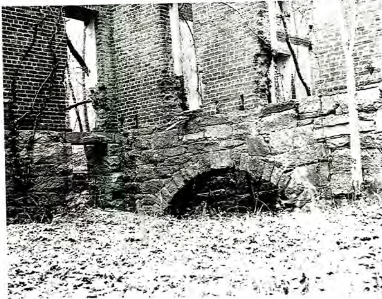
A. 9Ge37. Main factory building, east addition from Southeast.
