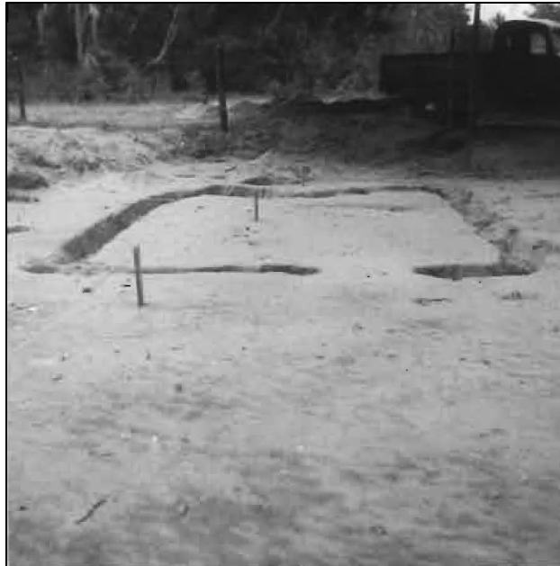
Figure 37. View of Structure 5. Note doorway at right center.
