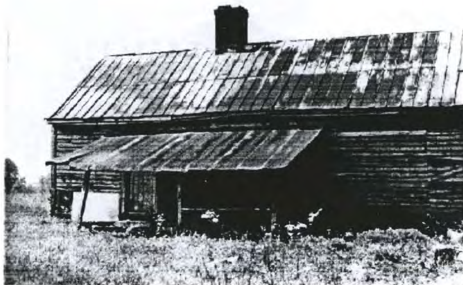
Barton-Swift-Nolan House-Structure 1-Kitchen wing looking south.
