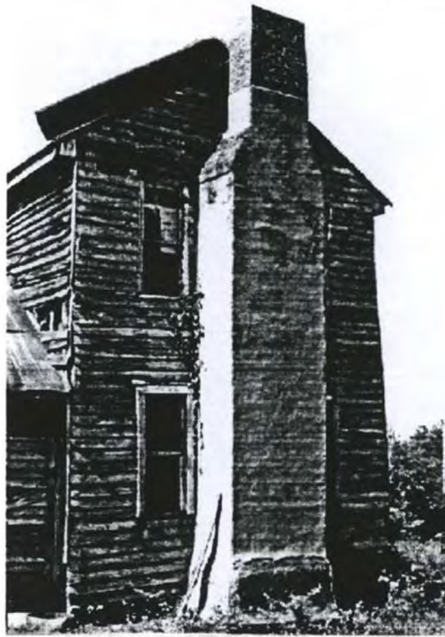
Barton-Swift-Nolan House-Structure 1-North end wall showing chimney with stucco.
