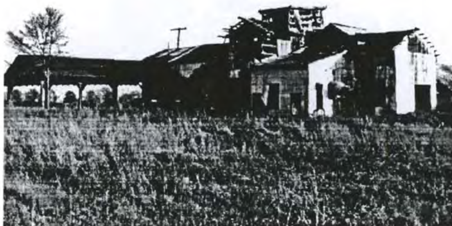
Nolan Plantation-Structure 16-Cotton gin. View from the northwest.
