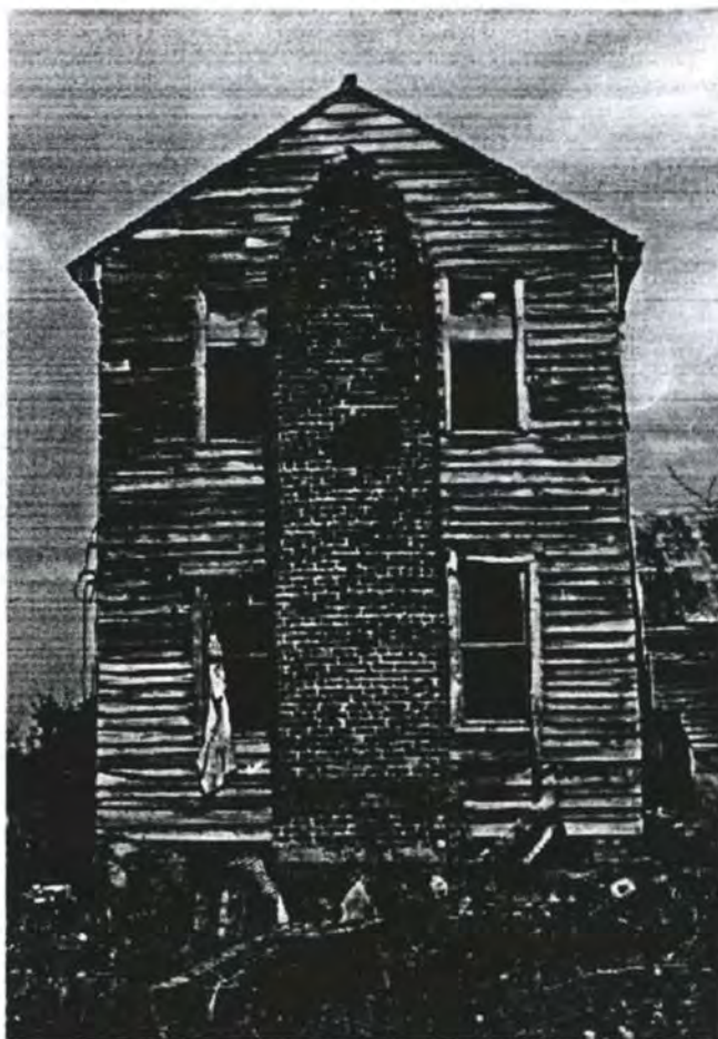
Barton-Swift-Nolan House-Structure 1-South end wall.
