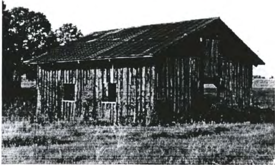
Nolan Plantation-Structure 15-Barn behind cotton gin. View from the southeast.
