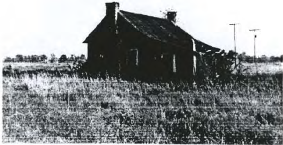
Nolan Plantation-Structure 7-tenant house, looking southeast. This house faces Georgia highway 83.
