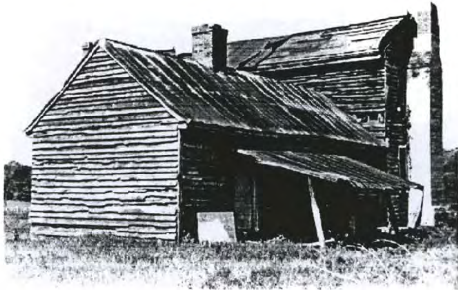
Barton-Swift-Nolan House-Structure 1-Kitchen wing looking southwest.
