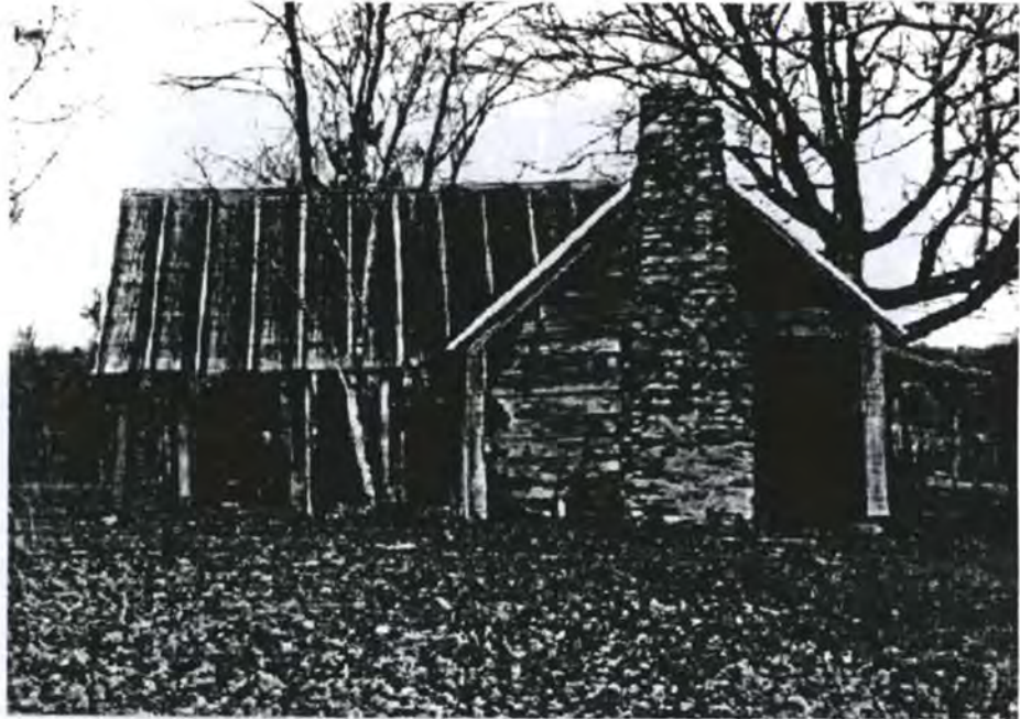
Nolan Plantation-Structure 3-log tenant house, south wall.
