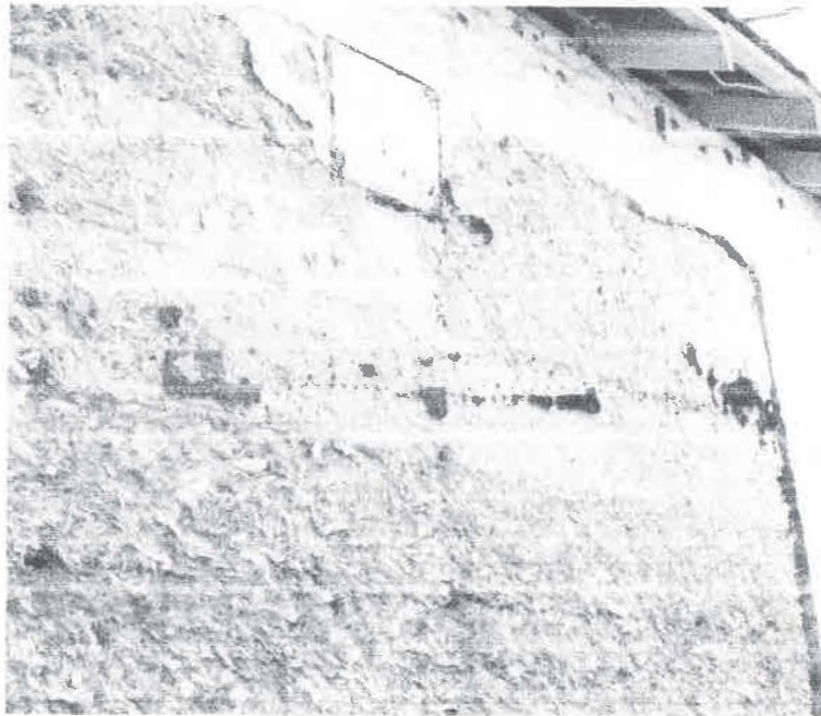
A bricked in vent near the roofline on the west wall and remnants of flashing and nails from a roof for a no longer attached building are visible on the same wall.
