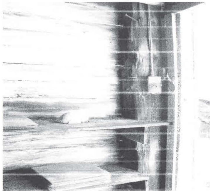
Tree trunk used as a building support and shelves on eastern wall of southeastern portion of wooden building
