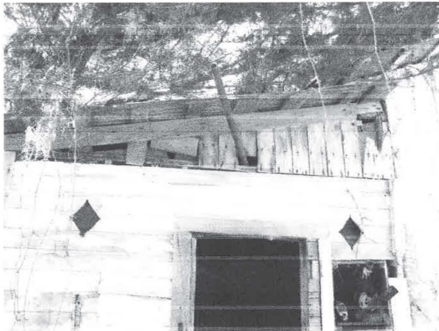
Northern "Power House" Elevation where Roofline shows signs of decay
