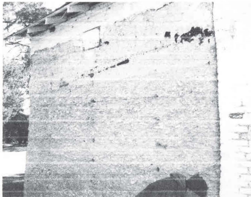
West tabby and brick wall joint as well as several courses of brick visible atop the older tabby
