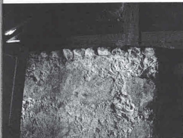
Photo. 1147. Interior of north tabby's north elevation. Close-up of sand bricks.
