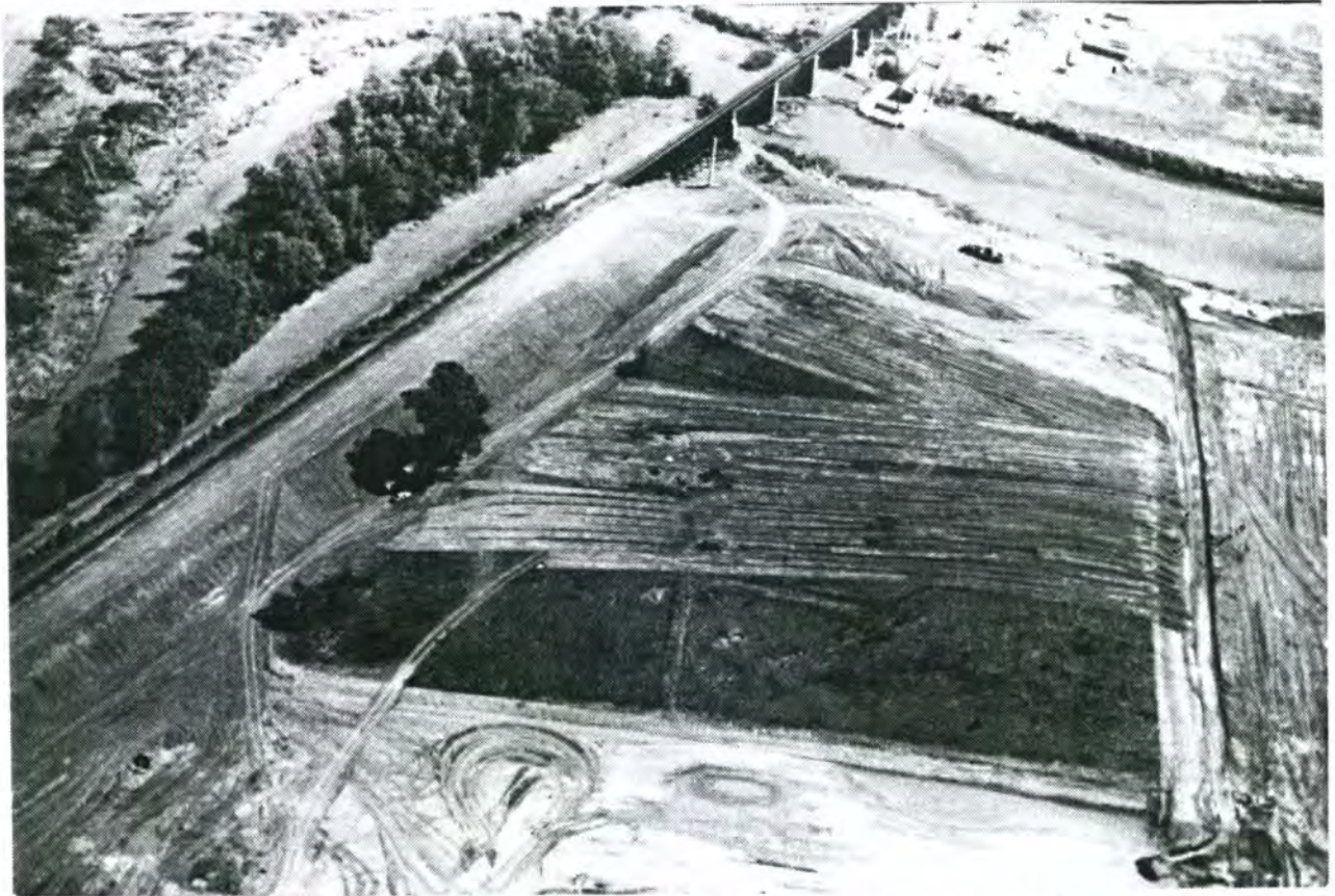
Plate 1 - Aerial View, Initial Excavations, 1977
